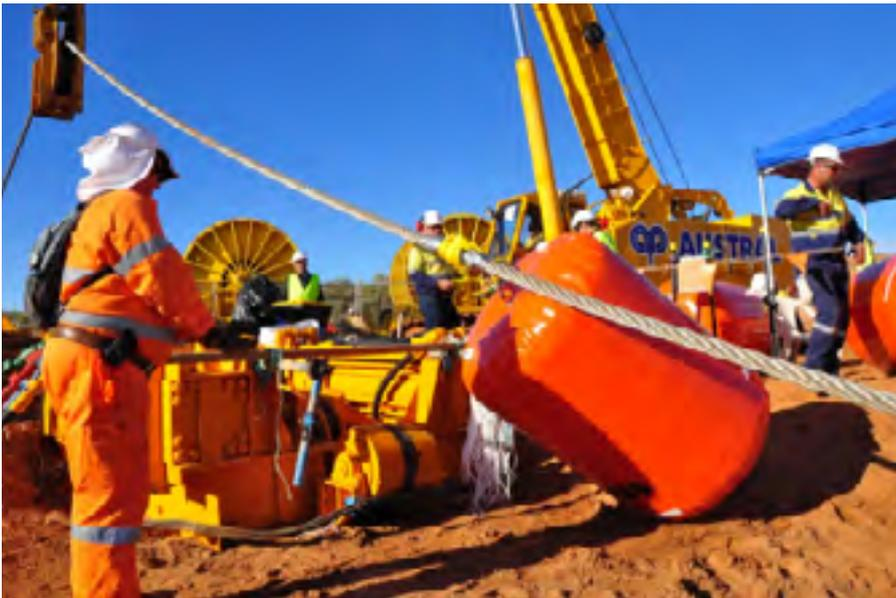
Fig 1: Seaflex 1t MBUs on Macedon shore pull head cable, 2012
