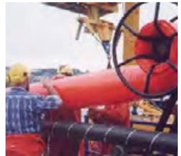
2. SeaSerpent being attached to the HVAC cable showing Seaflex manual brake DRS.
